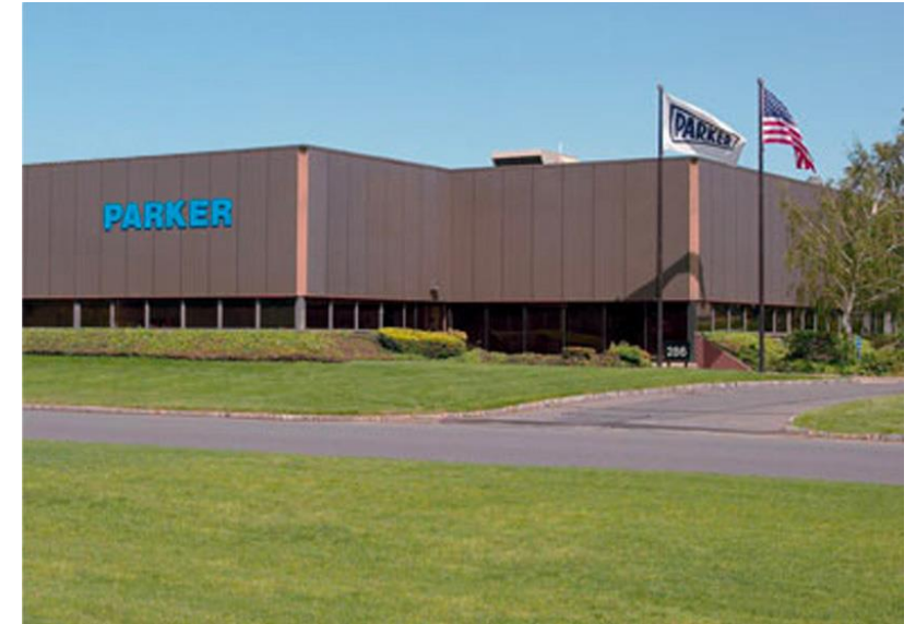
Parker Laboratories Inc. Headquarters, Fairfield, New Jersey
